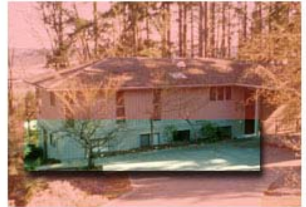
Inside ADU - lower level.
