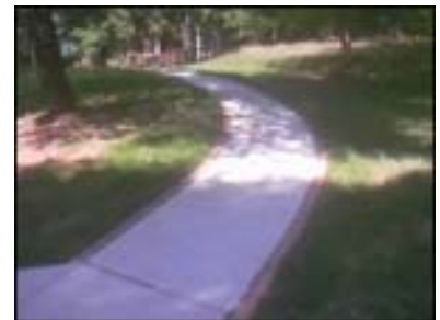
Springfield Oaks HOA Accessible Path
